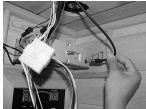
FIG-21 Link the antenna connectors
