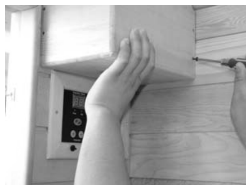
FIG-22.1 Fix the CD player back cover with screws
