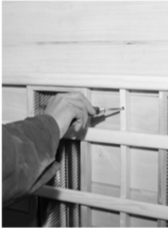
FIG-11 Assembling sitting board
