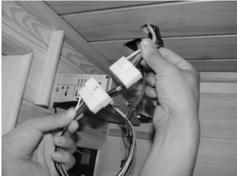
FIG-18 Link the CD connectors
