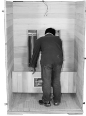
FIG-8 Assembling sitting board's support
