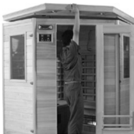
FIG-13 Assembling the inner top board
