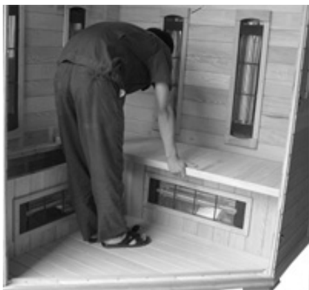
FIG-10 Assembling sitting board
