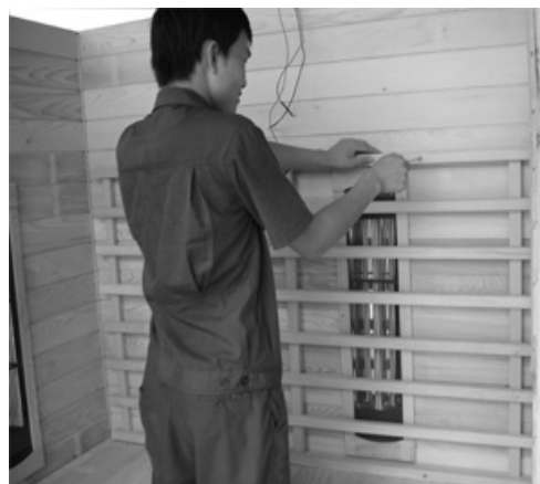
FIG-11 Fix the backrest with screws
