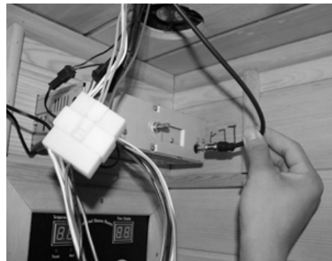
FIG-21 link the antenna connectors
