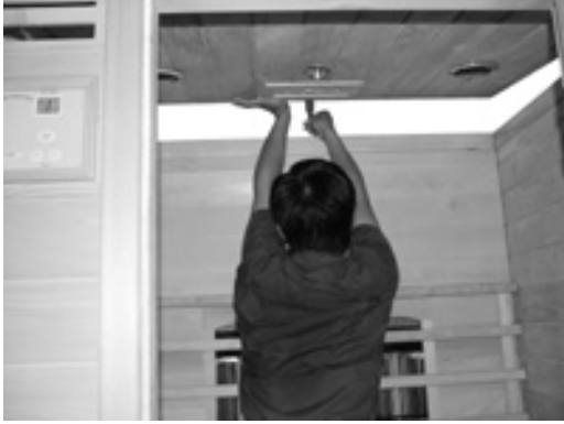
FIG-14 put through the wire
