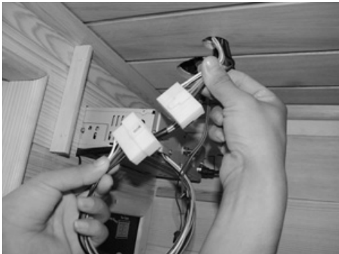
FIG-18 Link the CD connectors
