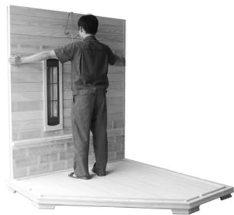
FIG-4 Assembling left back-side board
