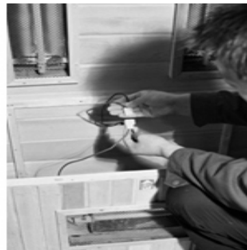
FIG-9 connecting the wire
