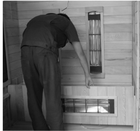
FIG-7 Assembling long sitting baffle
